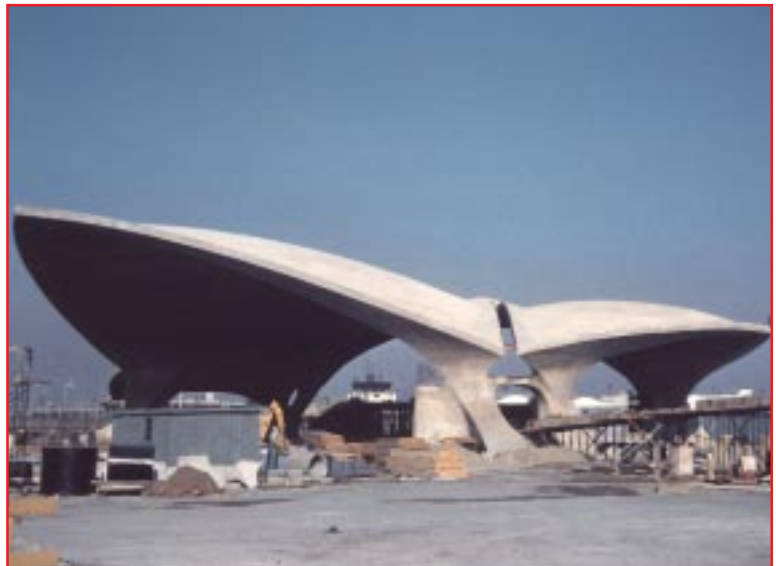
The old Idlewild control tower is visible in this picture of the cantilevered, concrete shell of what would become the TWA Flight Center. (Edgerton Aikman)
