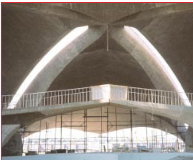
Also photographed during construction, the interior ceiling reveals skylights between the four roof sections. This view faces the street entrance to the terminal. (Alistair & Beverly Duncan)
