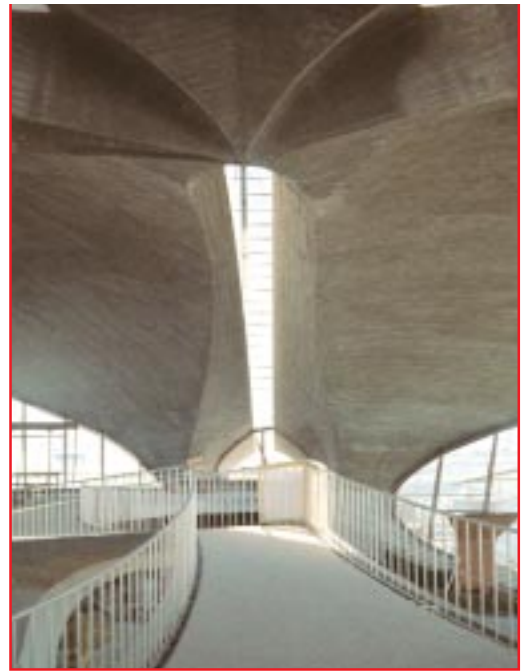
Facing airside, the upper walkway is naturally illuminated by a skylight in this photo taken shortly before construction was completed. The brushed-aluminum railings were designed to present a graceful pattern throughout the building. (Alistair & Beverly Duncan)
